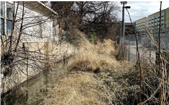
Boise City Canal, Before Project | Photo Source: CCDC
