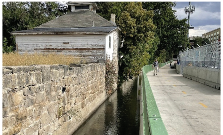
Boise City Canal Multi-Use Pathway, After Project | Source: CCDC
