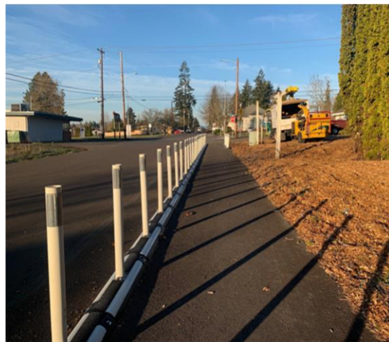
Flex Post SHUR CURB Separated Walkway: Extruded curbs or materials may be used to provide separated walkways or pathways on an interim basis or when stormwater treatment does not allow for traditional curb and gutter.
