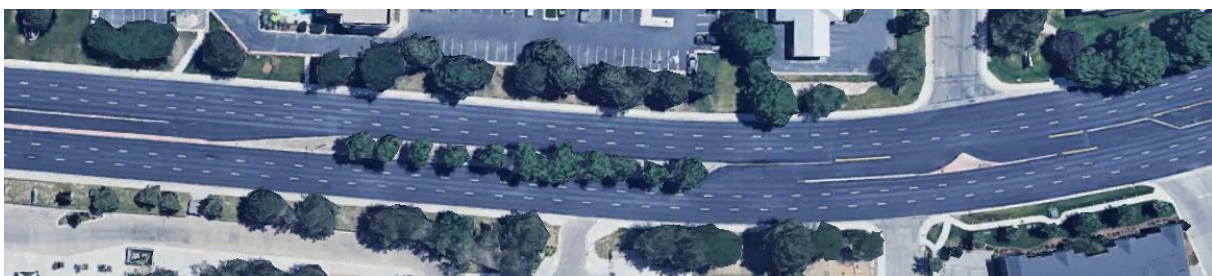
Raised Medians and Channelization on Parkcenter Boulevard in Boise: This treatment restricts left-turns from and channelized left-turns to adjacent side streets. Raised medians with larger buffer areas can provide a greater deterrent and are more visible than extruded curbs or other temporary treatments access management treatments. (Source: Google Maps)
