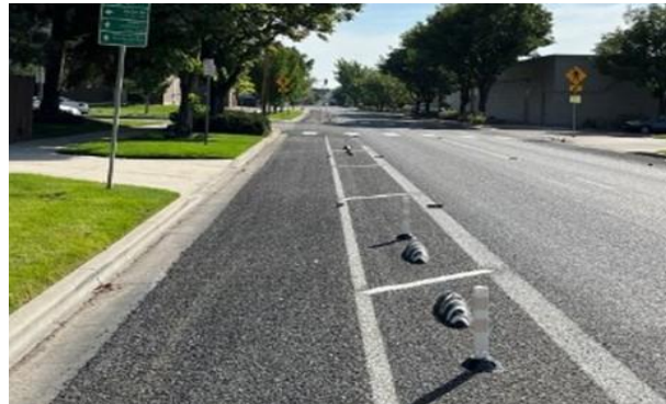
Protected Bike Lane with Temporary Delineation: Bollards or other vertical elements can be added to striping to provide a quick-build option for protected bike lanes.
