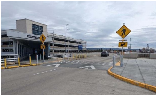
Example of Raised Crossing at Boise Airport: Raised crossings can increase awareness for drivers approaching a crossing and provide traffic calming benefits along a corridor, especially when placed at mid-block locations between roundabouts other traffic control devices. (Source: Google Maps)
