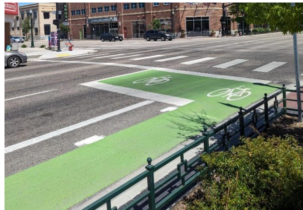
Example of Bike Box: Bike boxes increase the visibility of bicyclists and help to prevent conflict being left and right-turning vehicles and bicyclists. They are most typically used at signalized intersections with high-amounts of right and left-turning vehicles and can be implemented at a relatively low cost.
