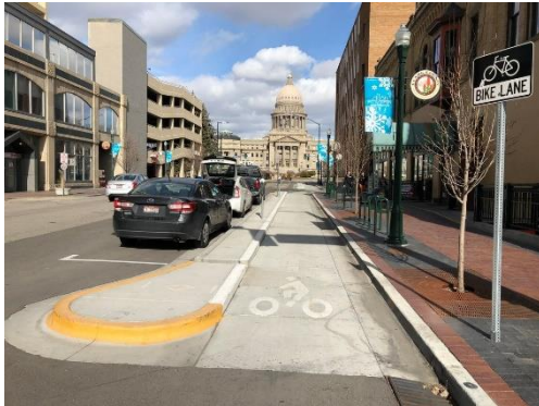
Protected Bike Lane: Vertical separation between the bike lane and travel lane provides a barrier between vehicles and people biking. This may be provided by curb, parking, or other vertical elements.
