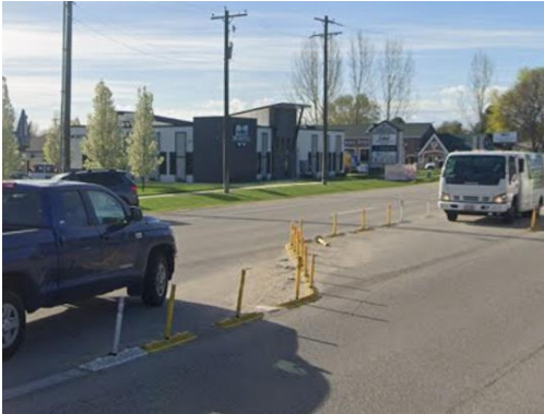
Access Management with Vertical Delineation: Bollards or other vertical elements can be added to striping to provide a quick-build option for restricting access to and from local roads or driveways (Source: Google Maps).
