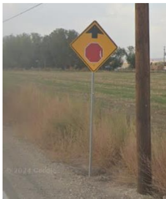
Advanced Warning Signage on Stop-Controlled Approach. (Source: Google Maps)
