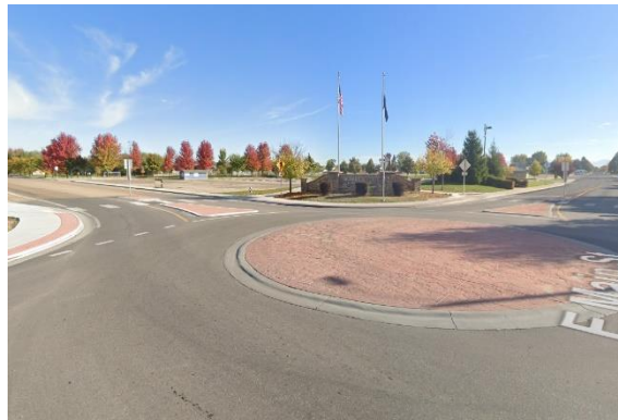
Example of Mini- Roundabout in Middleton: Mini-roundabouts can provide many of the safety and operational benefits while having a lower-cost, particularly in constrained, urban environments. Mini-roundabouts can also be implemented with quick-build materials for demonstration purposes. (Source: Google Maps)
