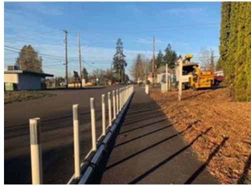
Flex Post SHUR CURB Separated Walkway: Extruded curbs or materials may be used to provide separated walkways or pathways on an interim basis or when stormwater treatment does not allow for traditional curb and gutter.
