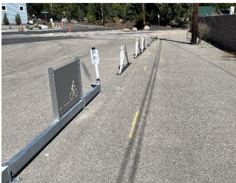
Protected Bike Lane with Temporary Delineation: Bollards or other vertical elements can be added to striping to provide a quick-build option for protected bike lanes.
