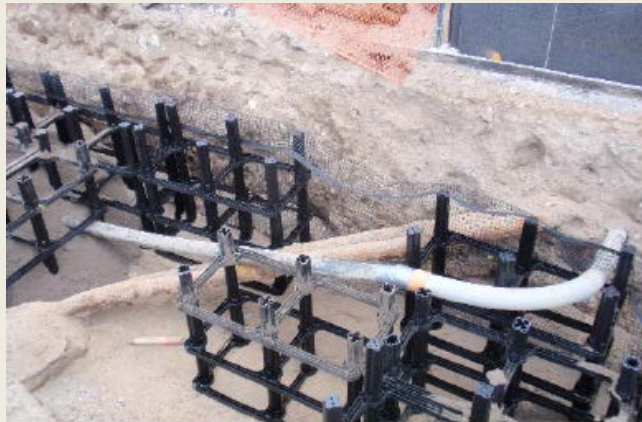
Silva Cells accommodate new and existing utilities.
