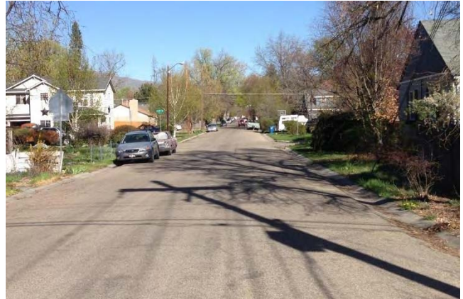
Many Local Streets Outside the North End Neighborhood Do Not Have Sidewalks
