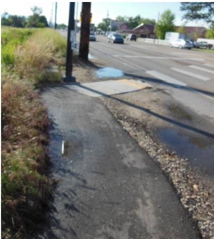
NE corner Bogart Ln and State St (No Sidewalks)
