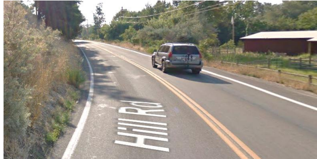
Hill Rd Looking Southeast (Narrow Shoulders, No Sidewalk, Limited Visibility)
