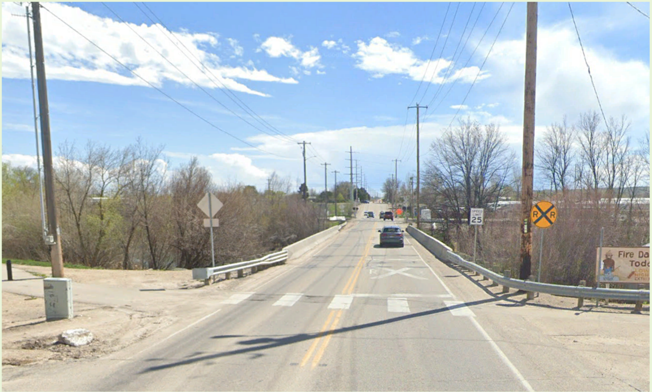
Figure 4 – Existing Condition over Swan Falls Bridge
