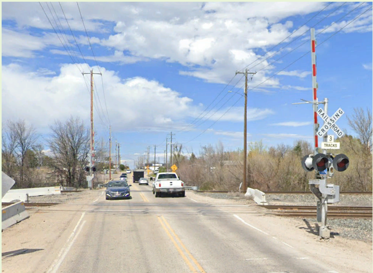
Figure 3 – Existing Conditions at Rail Crossing
