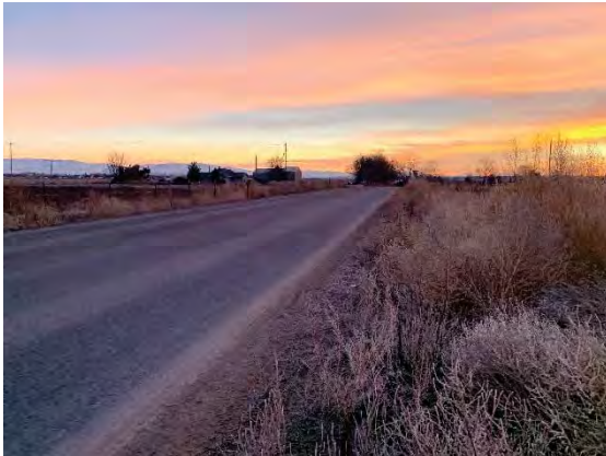
Looking east along Ardell Road
