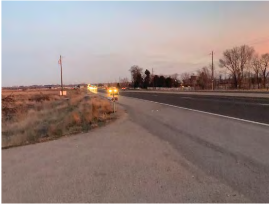
Looking north along Meridian Road
