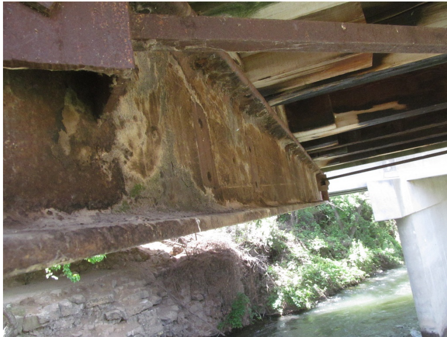
Photo 17: FB 3 – Holes and Different Cross Bracing Connection
