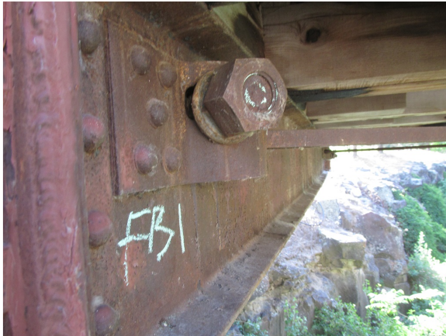
Photo 15: Lower Cross Bracing through FB 1
