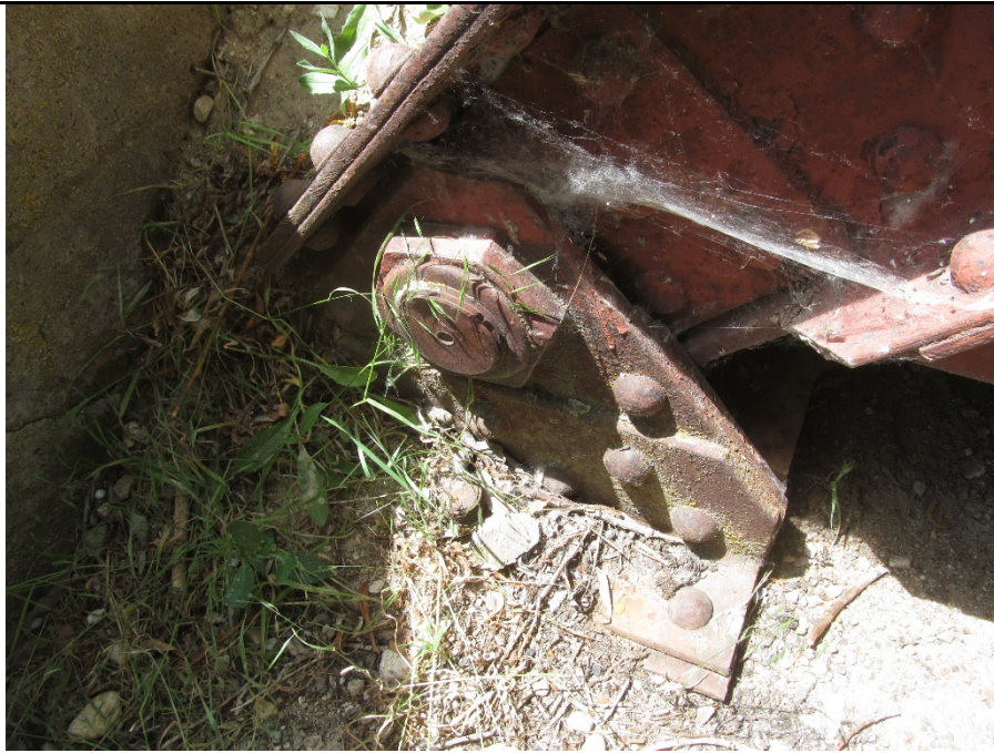
Photo 23: Fixed Bearing at Abutment 2
