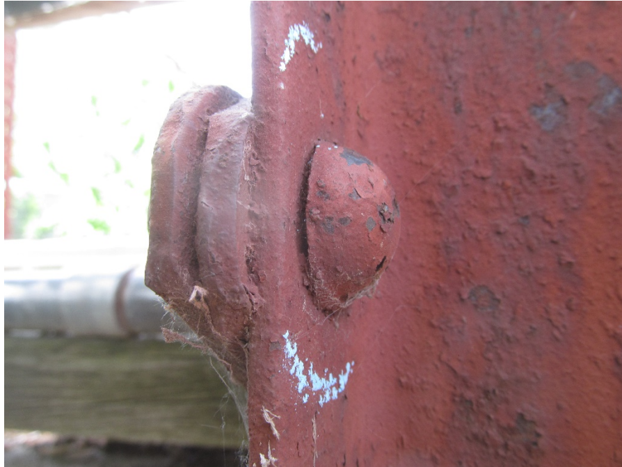
Photo 3: Pack Rust Forming Under Rivet Head
