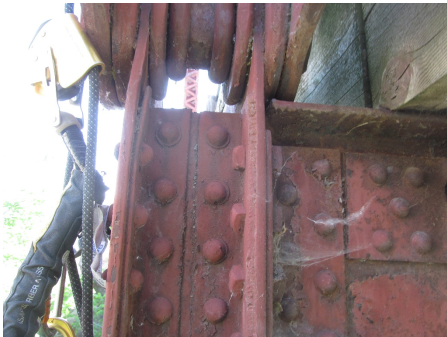
Photo 18: Out of Alignment Floor Beam Connection at L5B and FB 2
