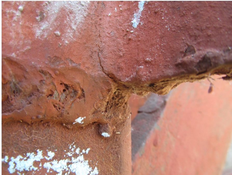
Photo 11: Cracked weld on the Outside of the Connection at L5A
