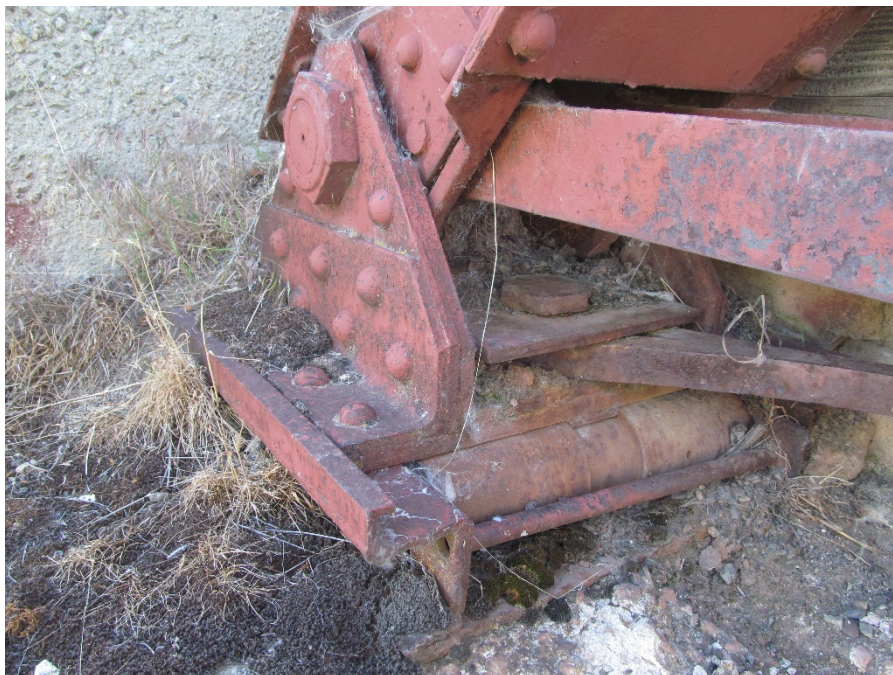
Photo 22: Moveable Bearing at Abutment 1
