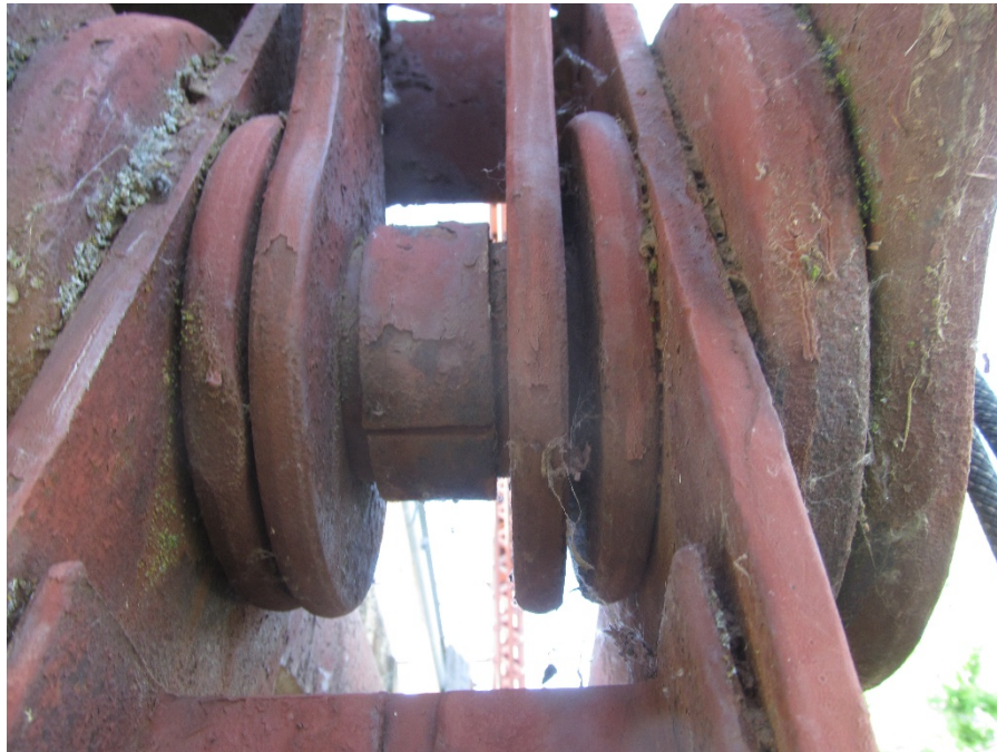
Photo 9: Undersized Eyebar Spacer at L5 and L9
