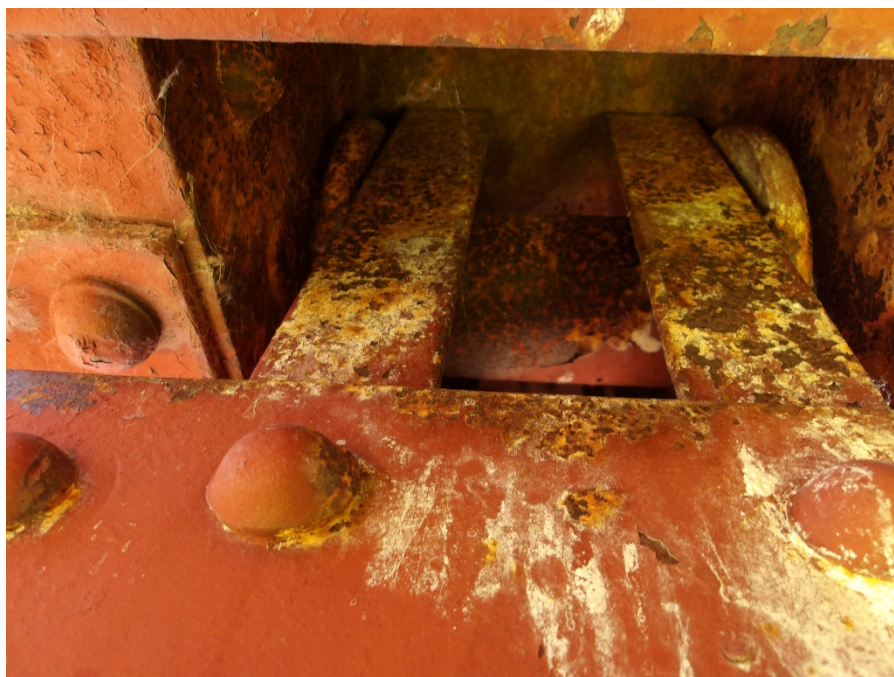
Photo 4: Surface Corrosion at U8A
