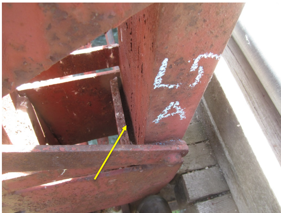
Photo 10: 1/2" Pack Rust between Vertical Truss Member and Welded Connection Plate at L5A
