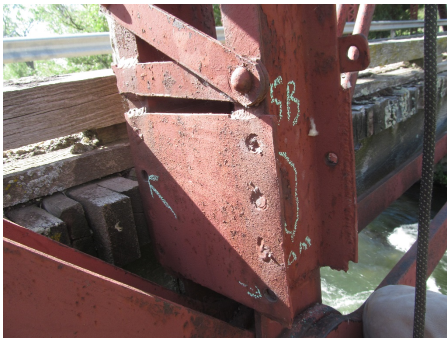
Photo 12: Welded Connection at L5B
