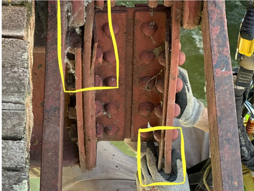
Photo 19: Typical Pack Rust Prying at Floor Beam to Vertical Connection
