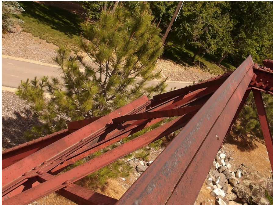
Photo 16: Bent Portal Bracing
