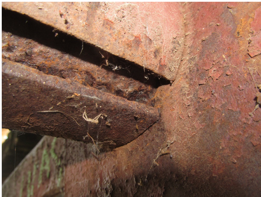
Photo 8: Pack Rust and Surface Pitting at the Lower Chord Pin
