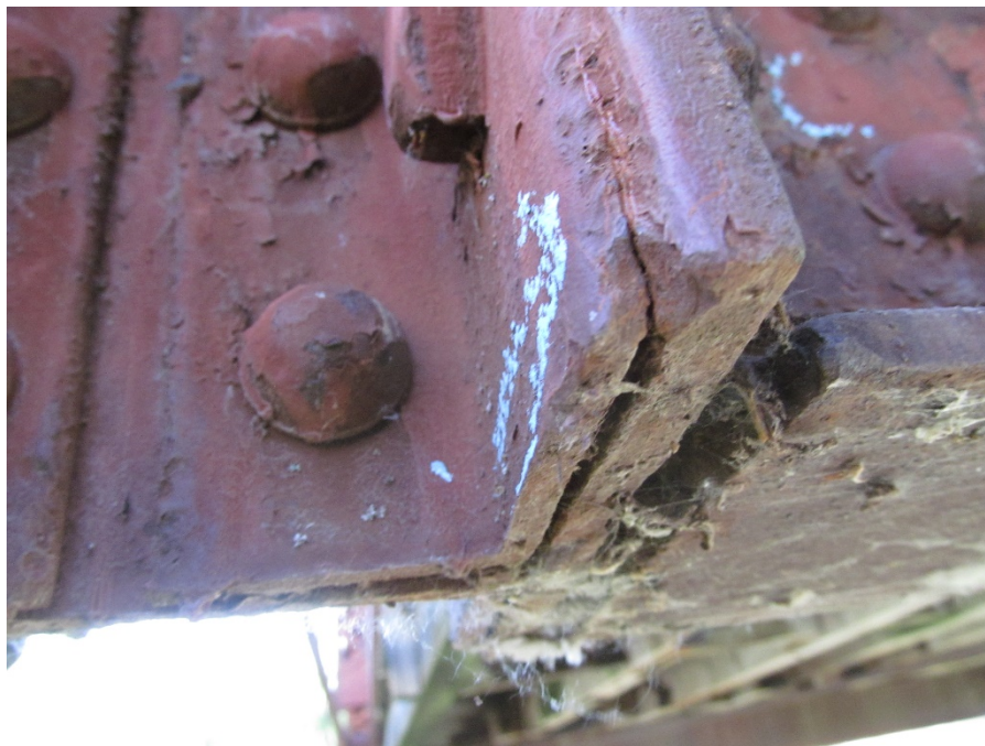
Photo 20: Cracked Weld Due to Pack Rust in Floor Beam to Vertical Connection at L5B
