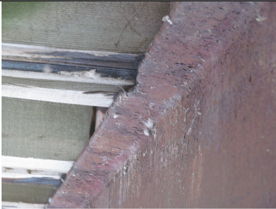
Photo 21: Missing Section from FB 2
