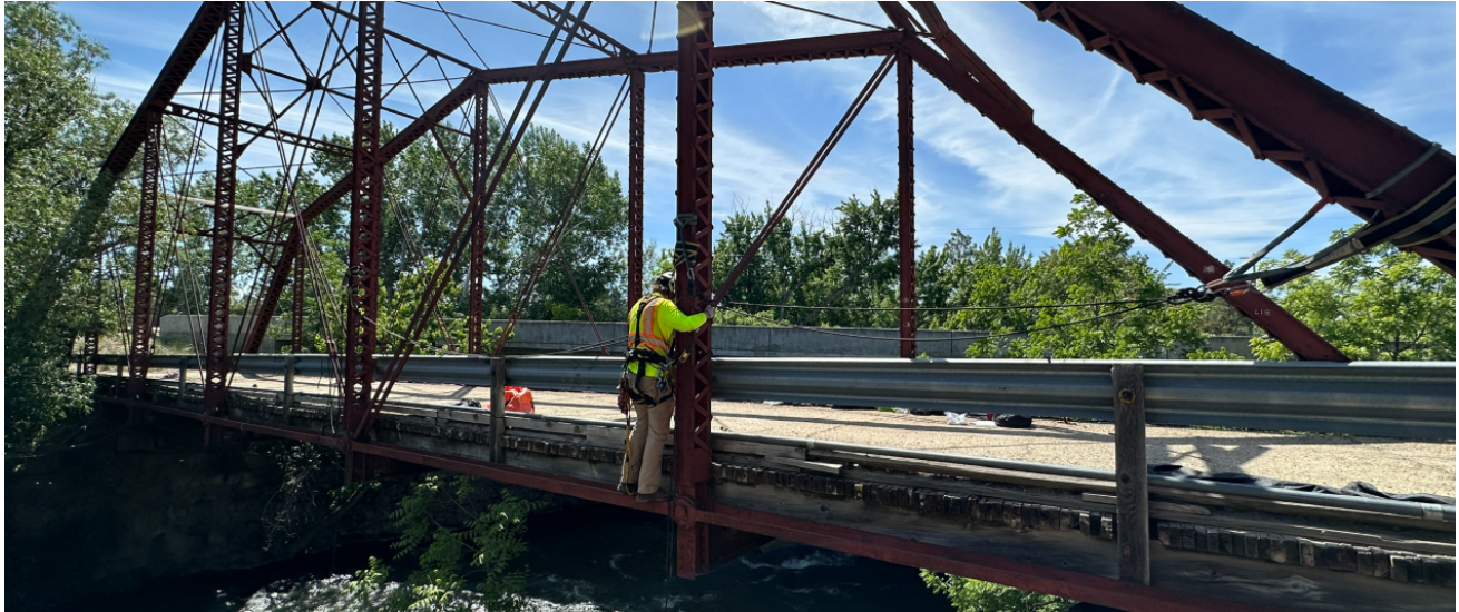
Figure 4: Inspection of Existing Steel Truss Bridge
