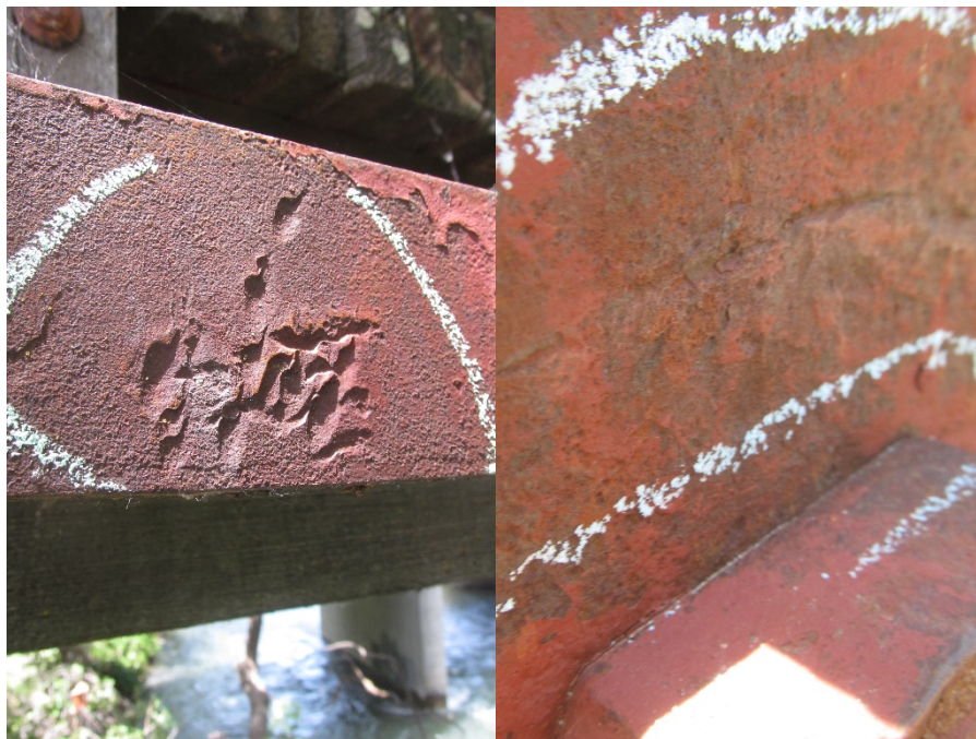
Photo 6: Surface Defects on Lower Chord Eyebar (L11AL12A Left, L5AL7A Right)
