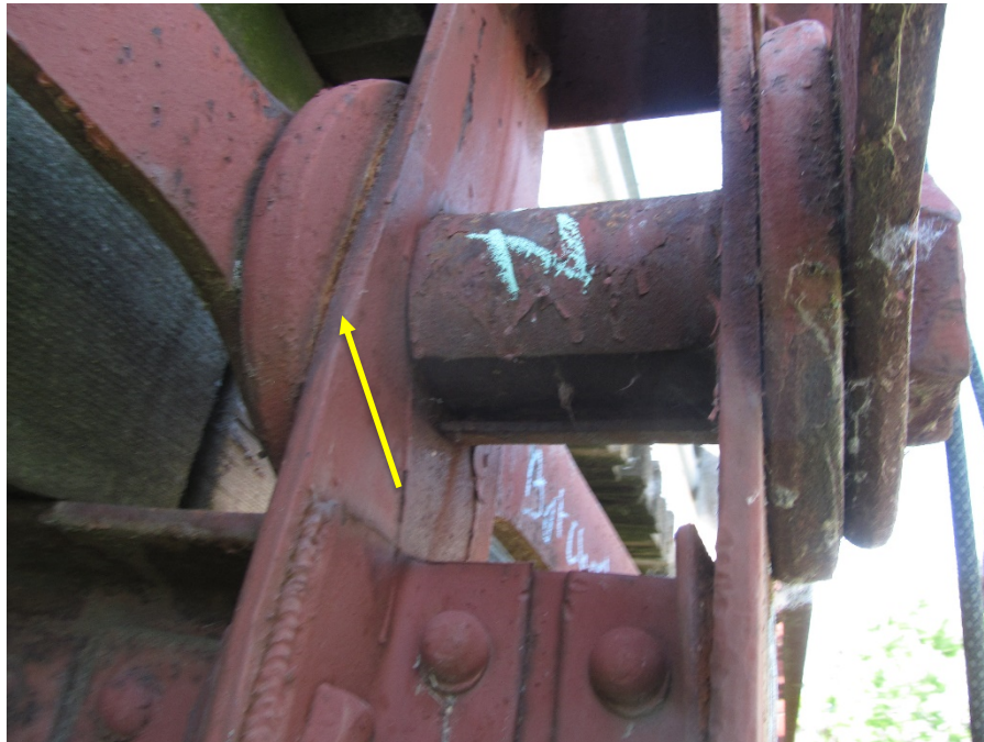
Photo 7: Pack Rust between Lower Chord Eyebar and Vertical Member
