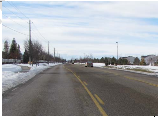
Road name and location: Birch Lane, Nampa Functional classification: Collector Function: Provides connection from local streets to arterial streets in the immediate area. Moderate length—generally less than one mile.
