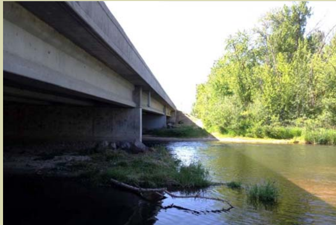
Eagle Road Bridge
