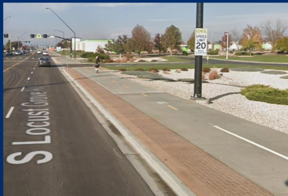
Shared-Use Path on Locust Grove Road (Source: Google Maps): Constructed in conjunction with Locust Grove Road widening after ACHD adoption of Livable Streets Performance Measures.
