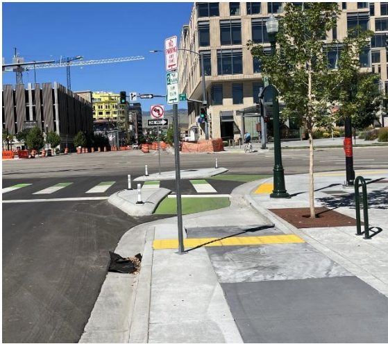
Example of Protected Intersection Elements: Protected intersections improve the comfort and safety of people walking and biking by reducing vehicle-turning speeds, reducing the speeds of people biking, and further separating people walking and biking from turning motor vehicles. They are typically used in conjunction with protected bike lanes on one or both intersecting streets; however, certain elements (e.g., reduced turning radii) can be applied at other intersections.
