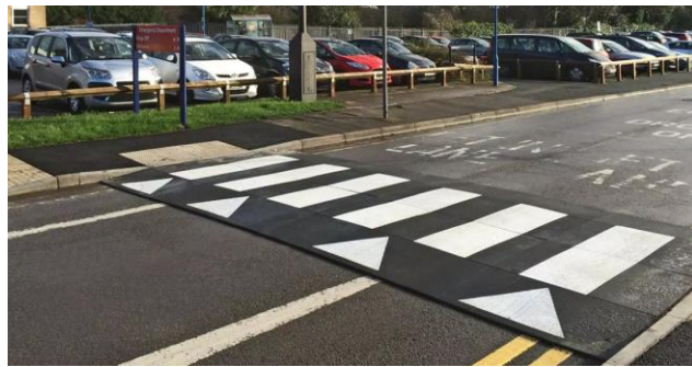
Example of Quick-Build Raised Crossing: Temporary raised crossing constructed of rubber or similar material can be used as a quick, low-cost alternative to permanent raised crossings. (Source: Rosehill Highways)
