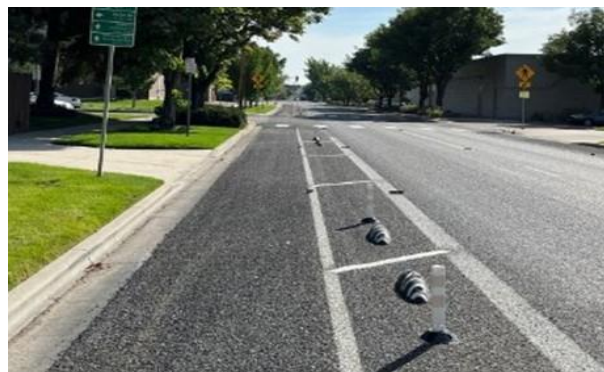
Protected Bike Lane with Temporary Delineation: Bollards or other vertical elements can be added to striping to provide a quick-build option for protected bike lanes.
