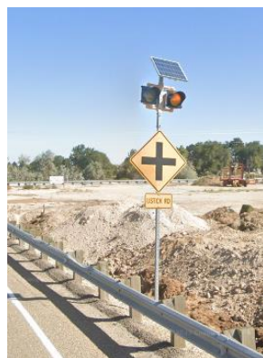
Advanced Warning Signage with Beacons on Through-Approach (Source: Google Maps)
