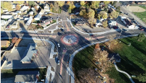
Single-Lane Roundabout at Linder and Main in Kuna
