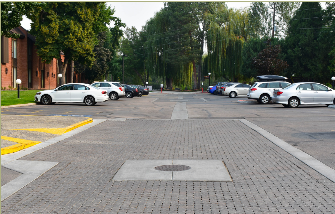
Figure 5. Permeable pavers at The Riverside Hotel
