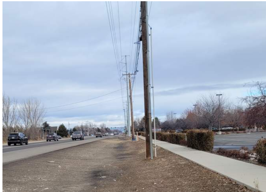
Figure 1-8 | Utility Poles Adjacent to Existing Sidewalk
