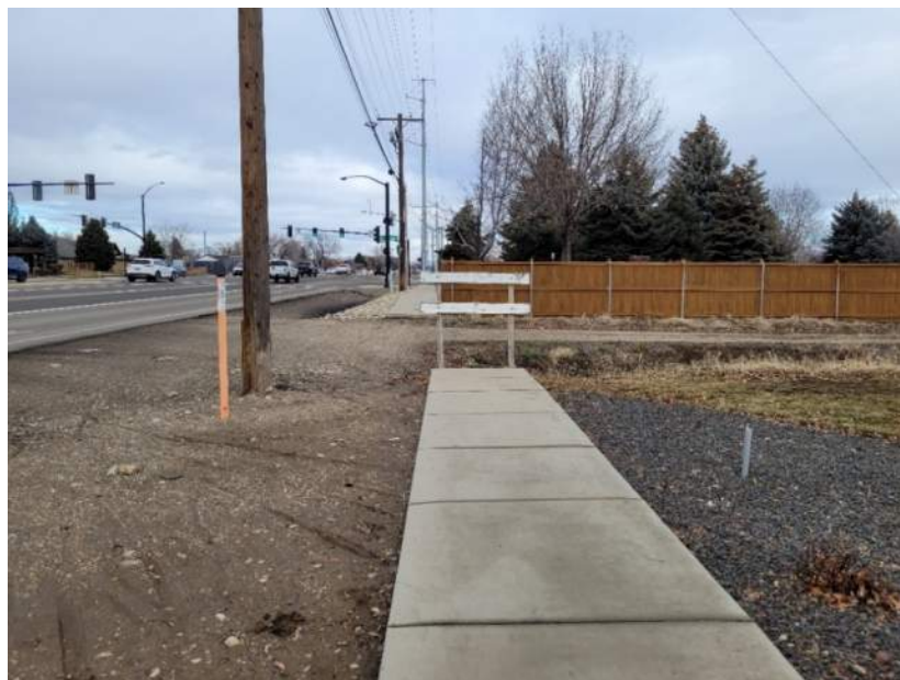
Figure 1-11 | Misaligned Sidewalk
