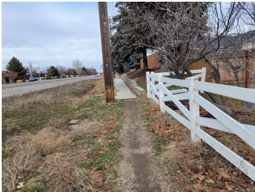
Figure 1-9 | Discontinuous Sidewalk
