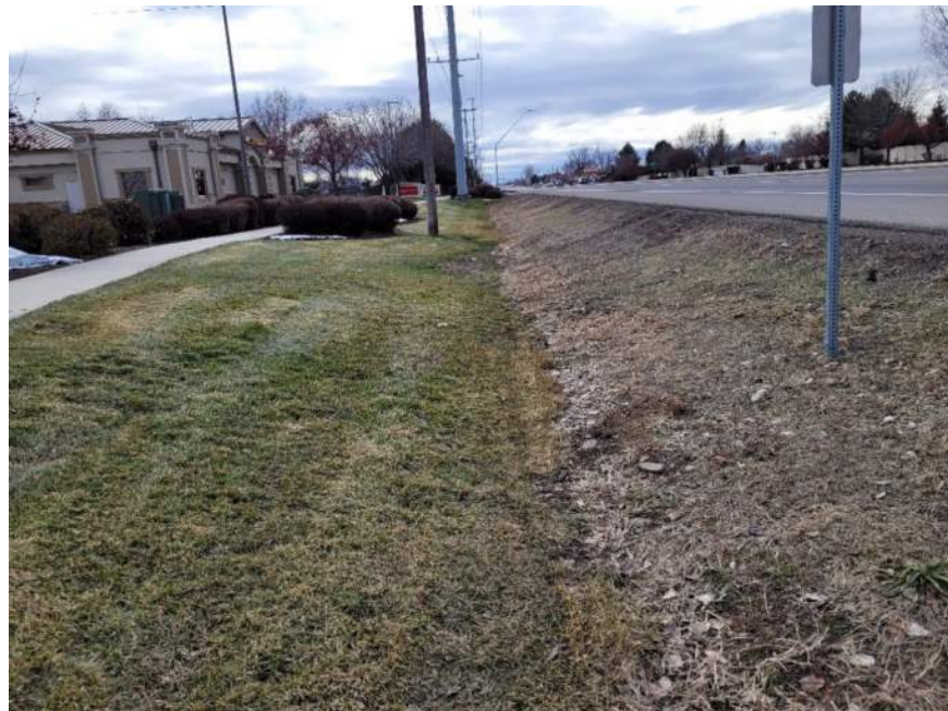
Figure 1-4: Existing Drainage Swale
