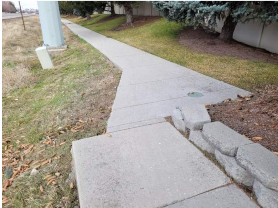
Figure 1-10 | Sidewalk Width Constriction
