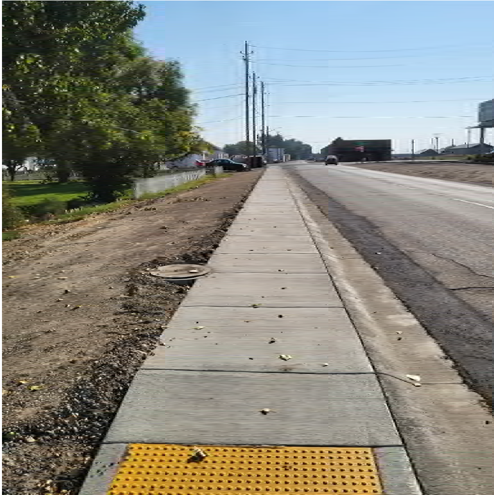
New Sidewalks in City of Wilder, 2022
