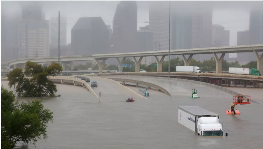
Interstate 45 inundated during Hurricane Harvey, August 2017.
