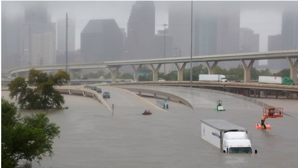
Interstate 45 inundated during Hurricane Harvey, August 2017.
