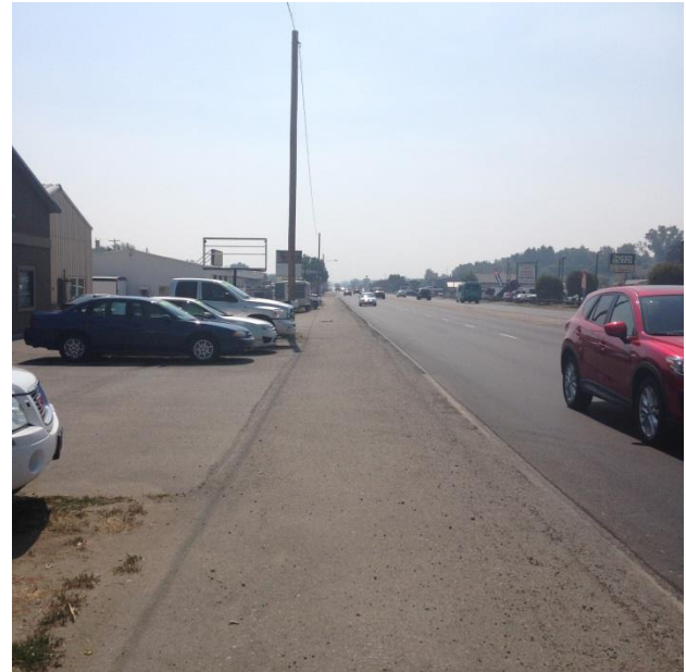
Existing shoulder with open access frontage on Chinden Boulevard east of 50 th Street
