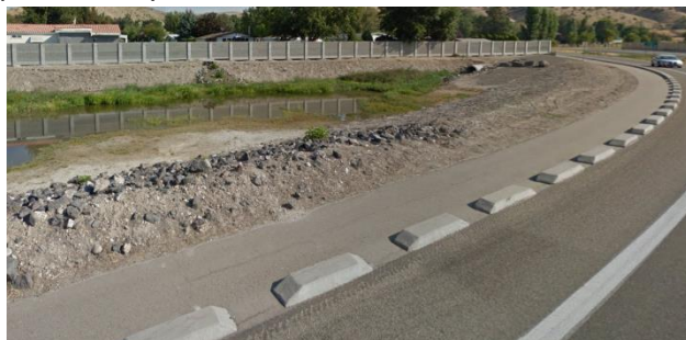
Extruded curb walkway section on Hill Road Image Source: Google Streetview
