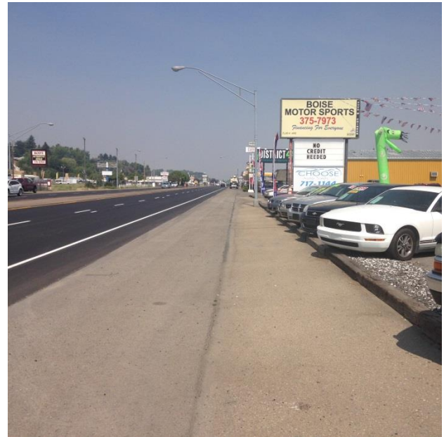
Existing shoulder on Chinden Boulevard west of 43 rd Street
