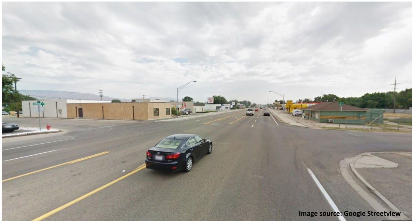
Figure 22 – 43 rd Street Intersection Existing Conditions (Looking East)
