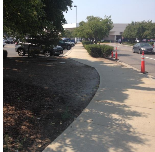
Existing sidewalk into Fred Meyer
