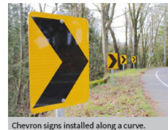
Chevron signs installed along a curve.
