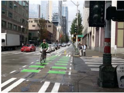
A Two-Way Protected Bike Lane Through Downtown
