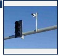
Project Description : Install upgraded signal controllers and radar detection at signalized intersections along the SH-55 (Eagle Road) corridor in Ada County that ties into ACHD's Signal Performance Measure software. The Signal Performance Measure software provides a visual display of traffic data to aid engineers in signal timing and coordination and assist technicians with better responsiveness for maintenance of field hardware.
