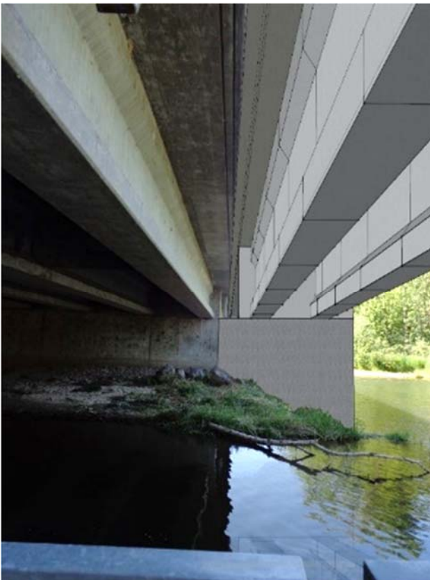
Photo 6 (Right): Rendering in photo showing proposed bike/ped bridge adjacent to existing bridge.
