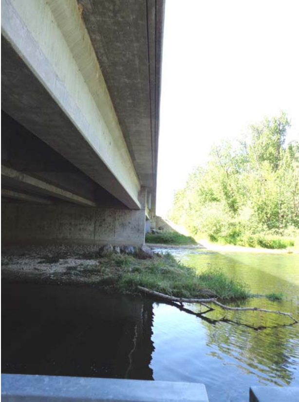
Photo 5 (Left): Existing Eagle Rd/SH-55 bridge, west side, looking south.
