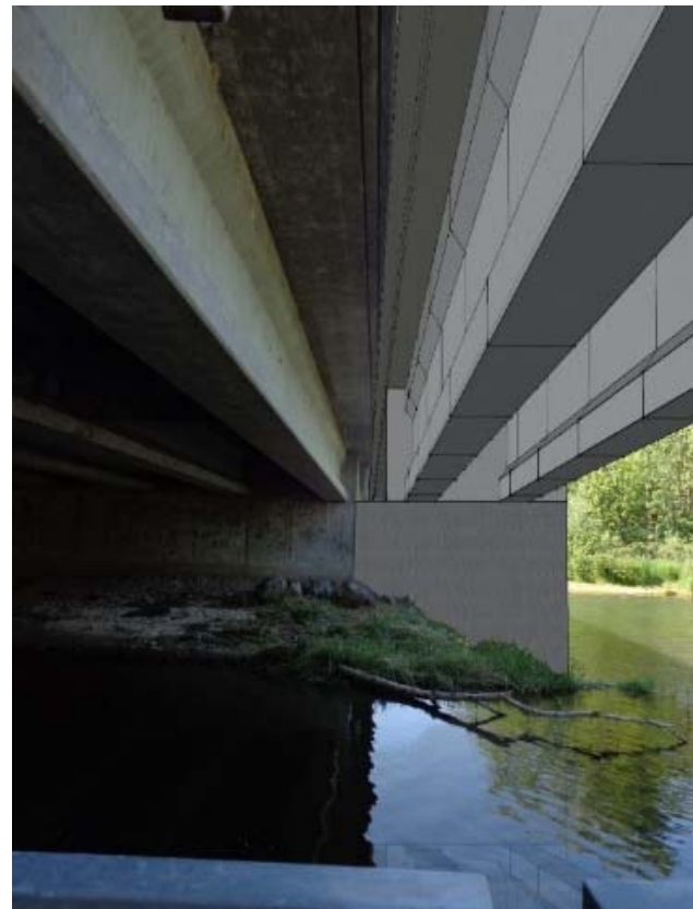
Figure 11: 'After' rendering (right) - concrete beams attached to existing bridge, looking under the west side of the bridge
