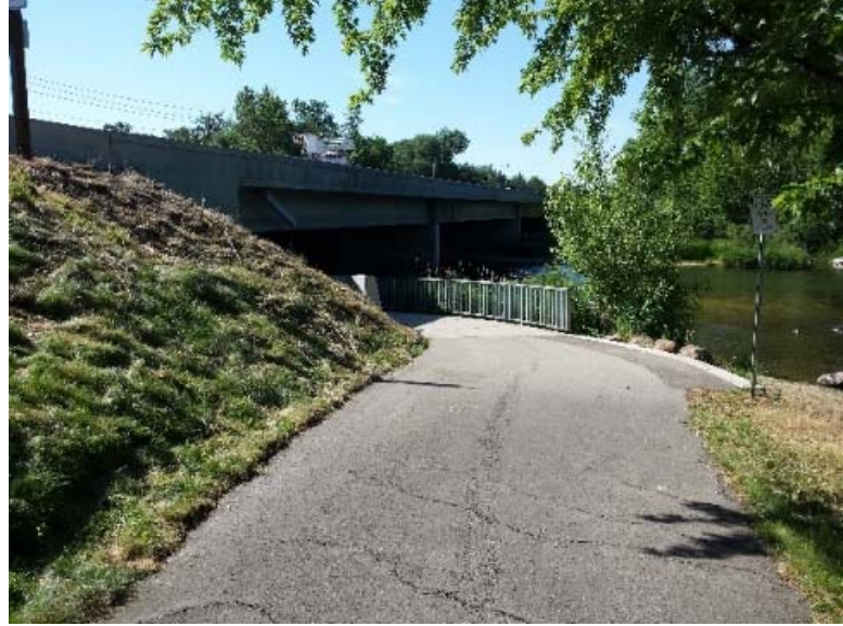
Figure 6: West side of SH-55 bridge, (June 2015) view looking at the NW corner "Point B" shown on Figure 4, "Bridge Plan View"
