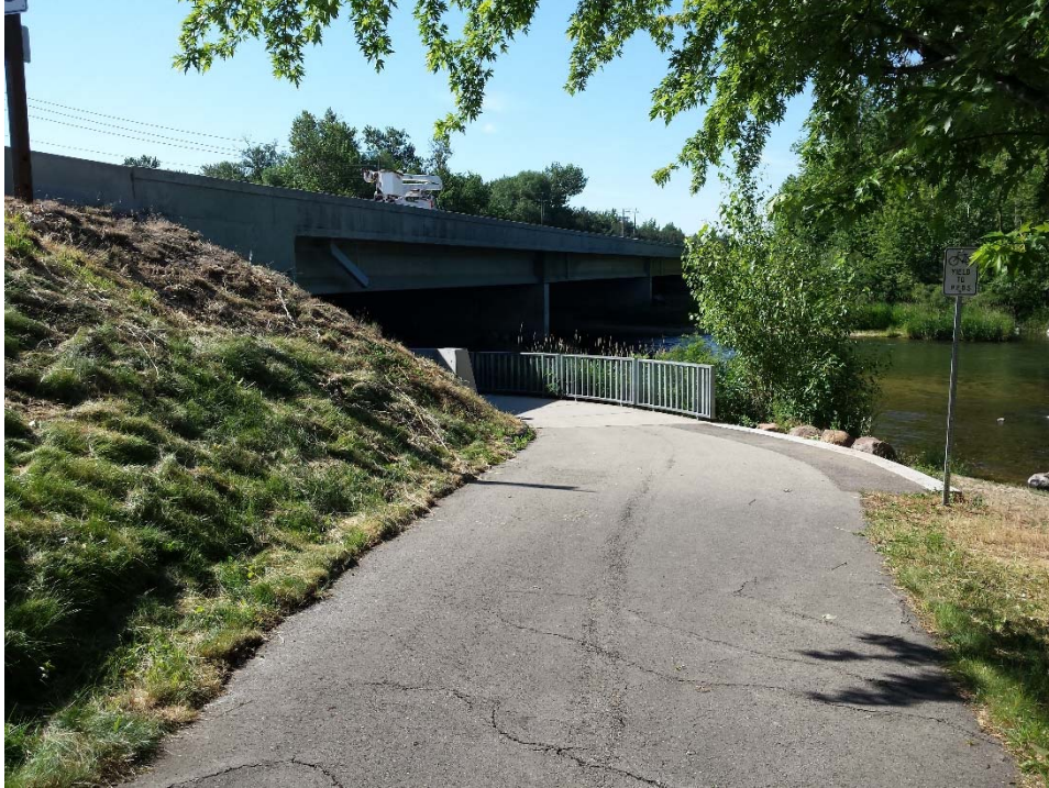
Photo 3 (Above): Existing Eagle Rd/SH-55 bridge, looking south/east at bike/ped underpass.
