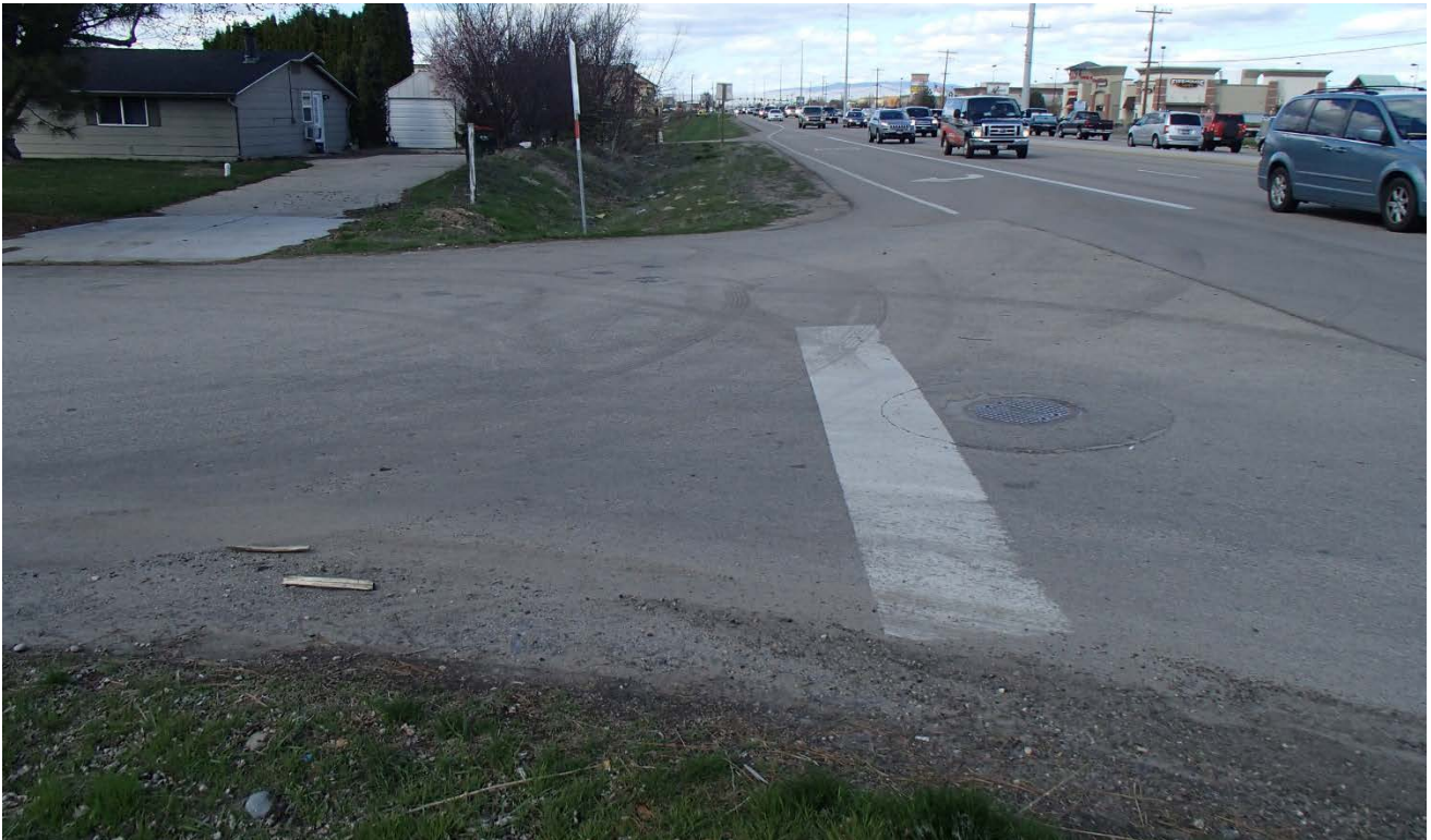
Looking north at the intersection of Eagle Road & Leslie Drive
