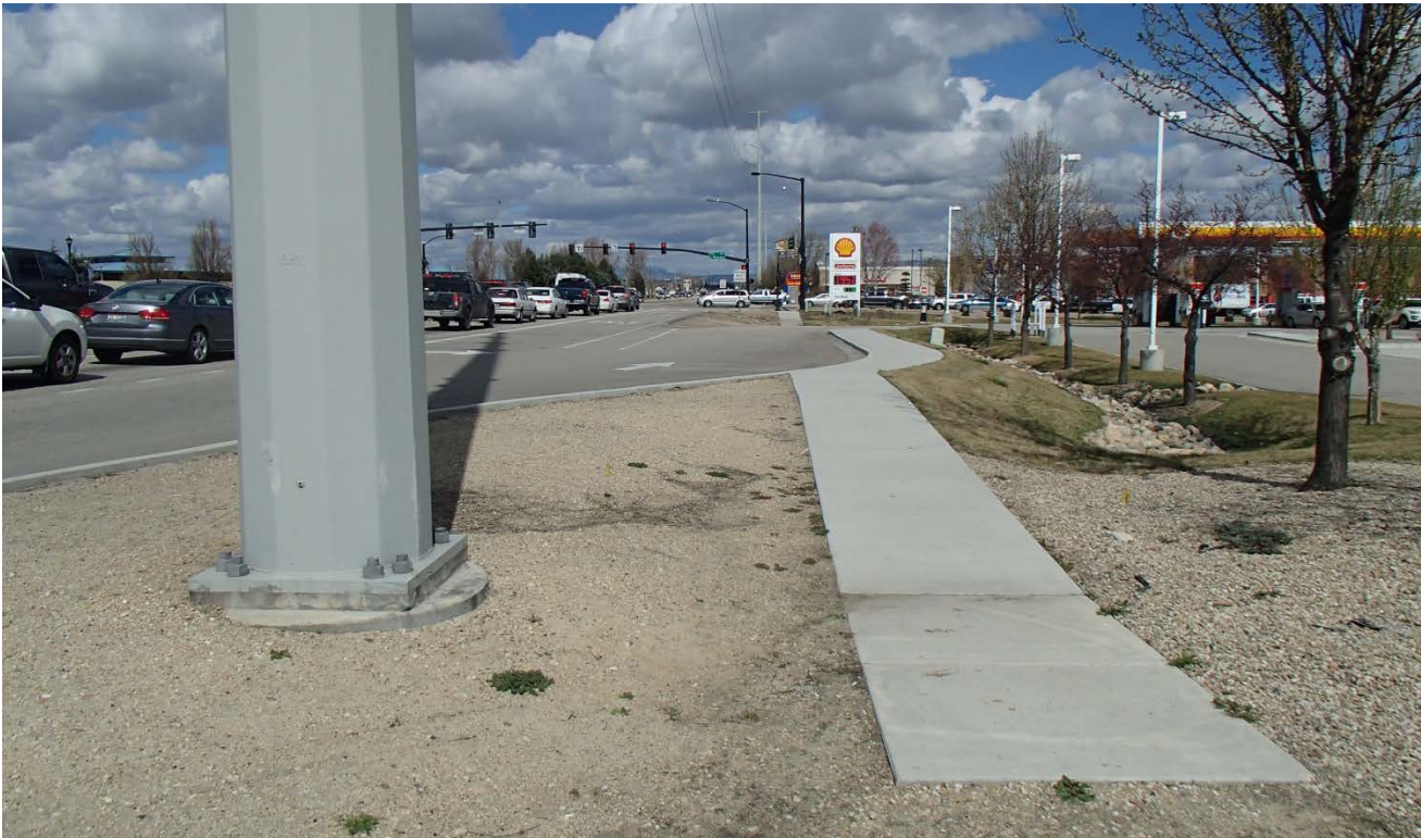
End of existing sidewalk adjacent to Shell gas station, looking north
