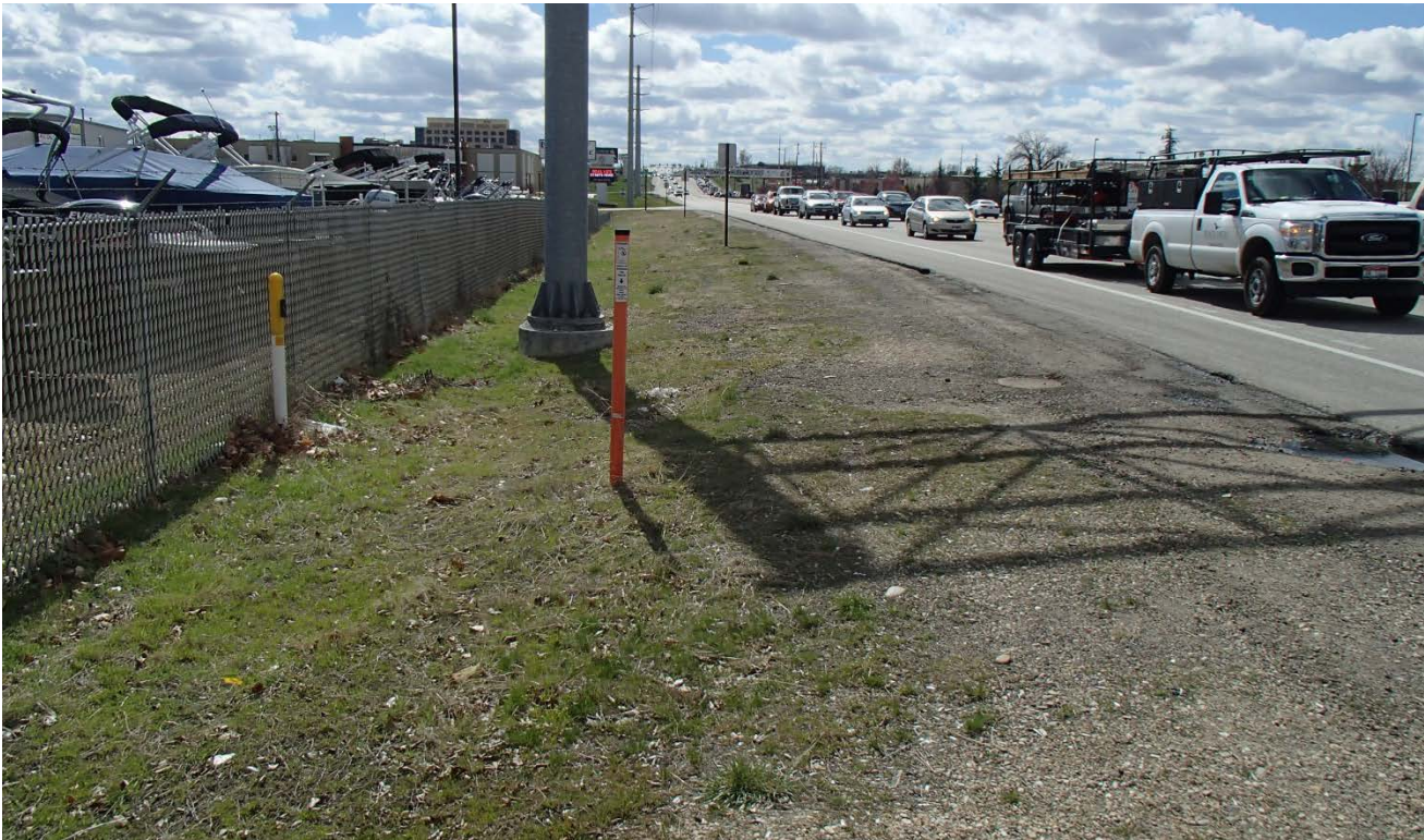
Looking south next to overhead sign over Eagle Road
