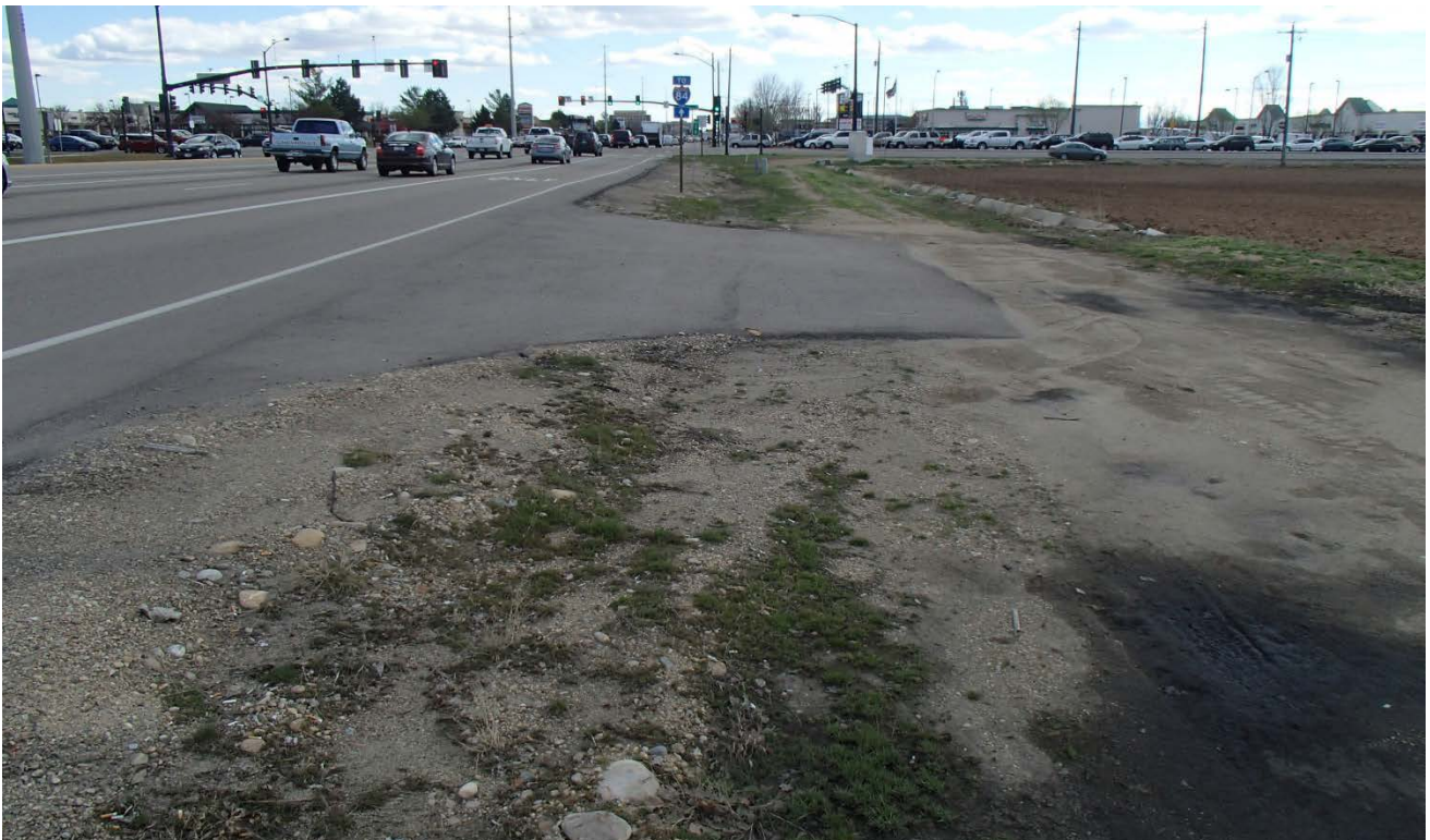
Looking south at the intersection Eagle Road & Fairview Avenue
