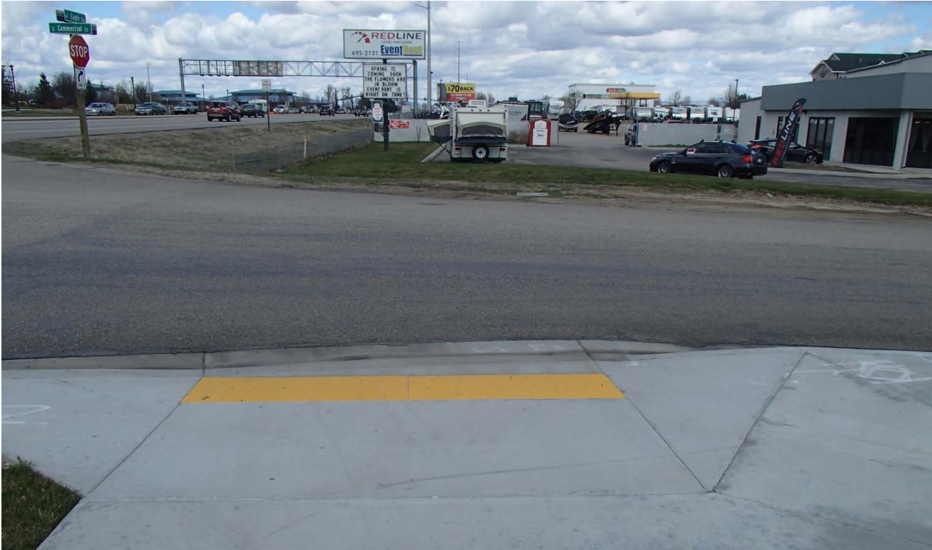
Looking north from end of existing sidewalk at Commercial Court
