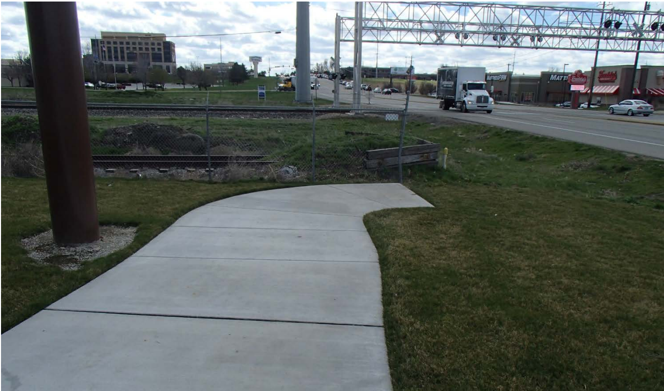
End of existing sidewalk north of railroad, looking south
