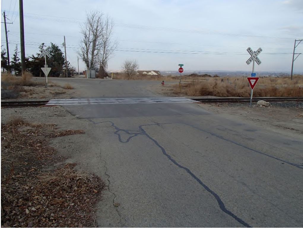
Figure 6 – Looking North at the Boise Valley Railroad Crossing
