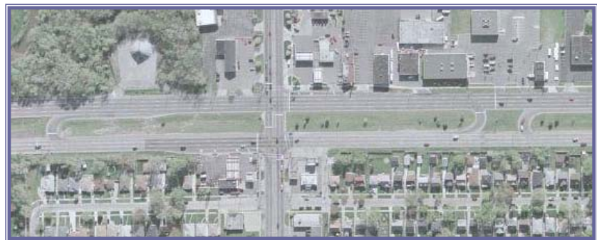
Figure 2-11: Aerial View of Median U-Turn Intersection
