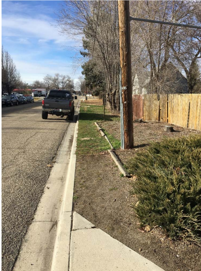
Figure 10. Missing Sidewalk on Roosevelt Avenue
