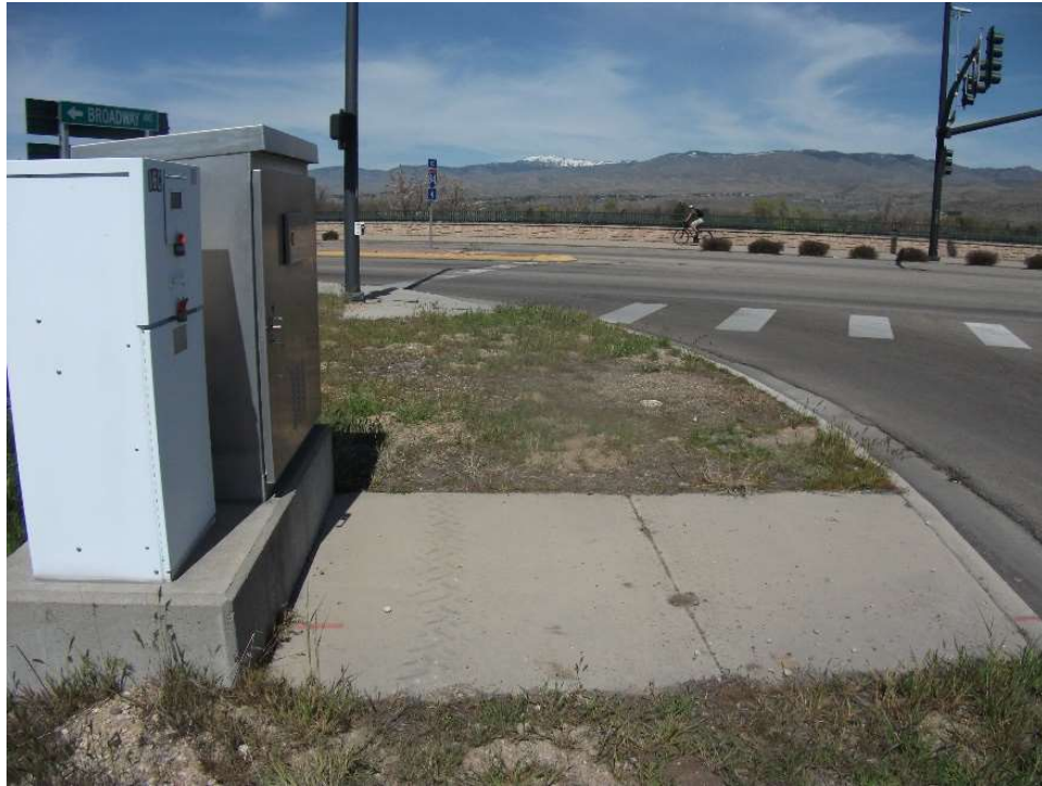
Alternative Route: Northbound Ramp & East Side of Broadway Constraint: Pedestrian Cross Walk with Light and Utility Box Relocation
