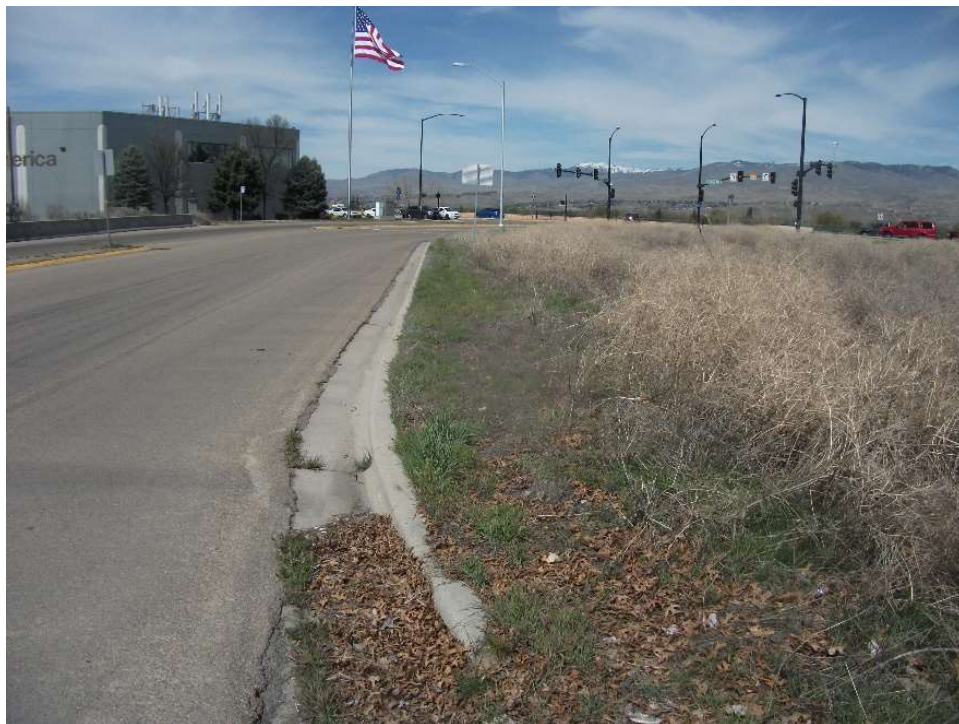
Alternative Route: Southbound Ramp & West Side of Broadway Constraint: Relocate Street Sign, Relocate Street Light
