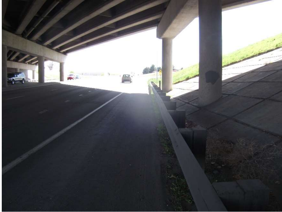
Alternative Route: Southbound Ramp & West Side of Broadway Constraint: Relocate Guard Rail, Relocate Street Lights
