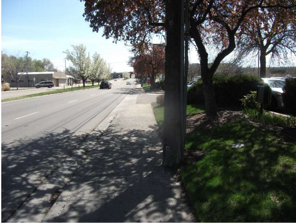
Alternative Route: Southbound Ramp & West Side of Broadway Constraint: Utilities Relocation, Tree and Landscaping Removal, Business Approach Intersection
