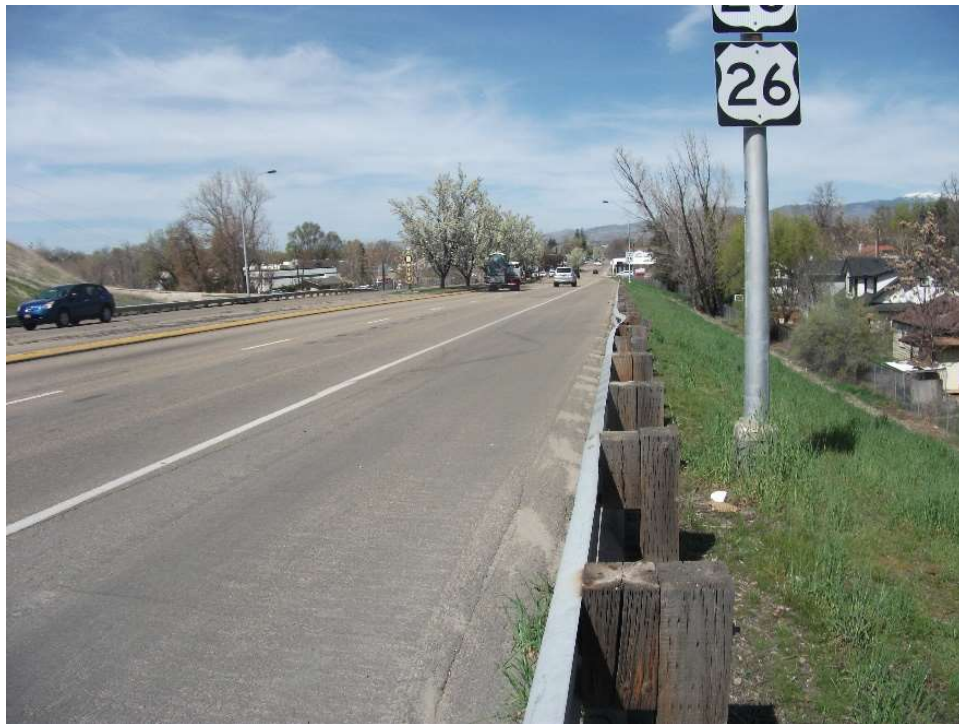
Alternative Route: Northbound Ramp & East Side of Broadway Constraint: Steep Embankment for Daylight Slopes
