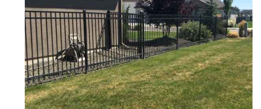
4 4 OR 5-FOOT HEIGHT OPEN VISION METAL FENCE NTS
