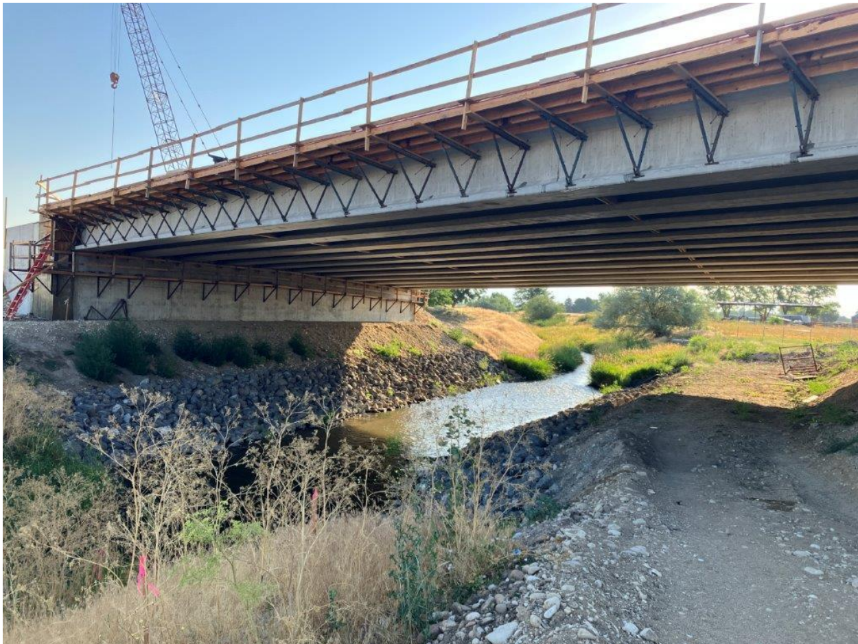
Figure 3 - SH-16 Ten Mile Creek Bridge Location (Looking East)
