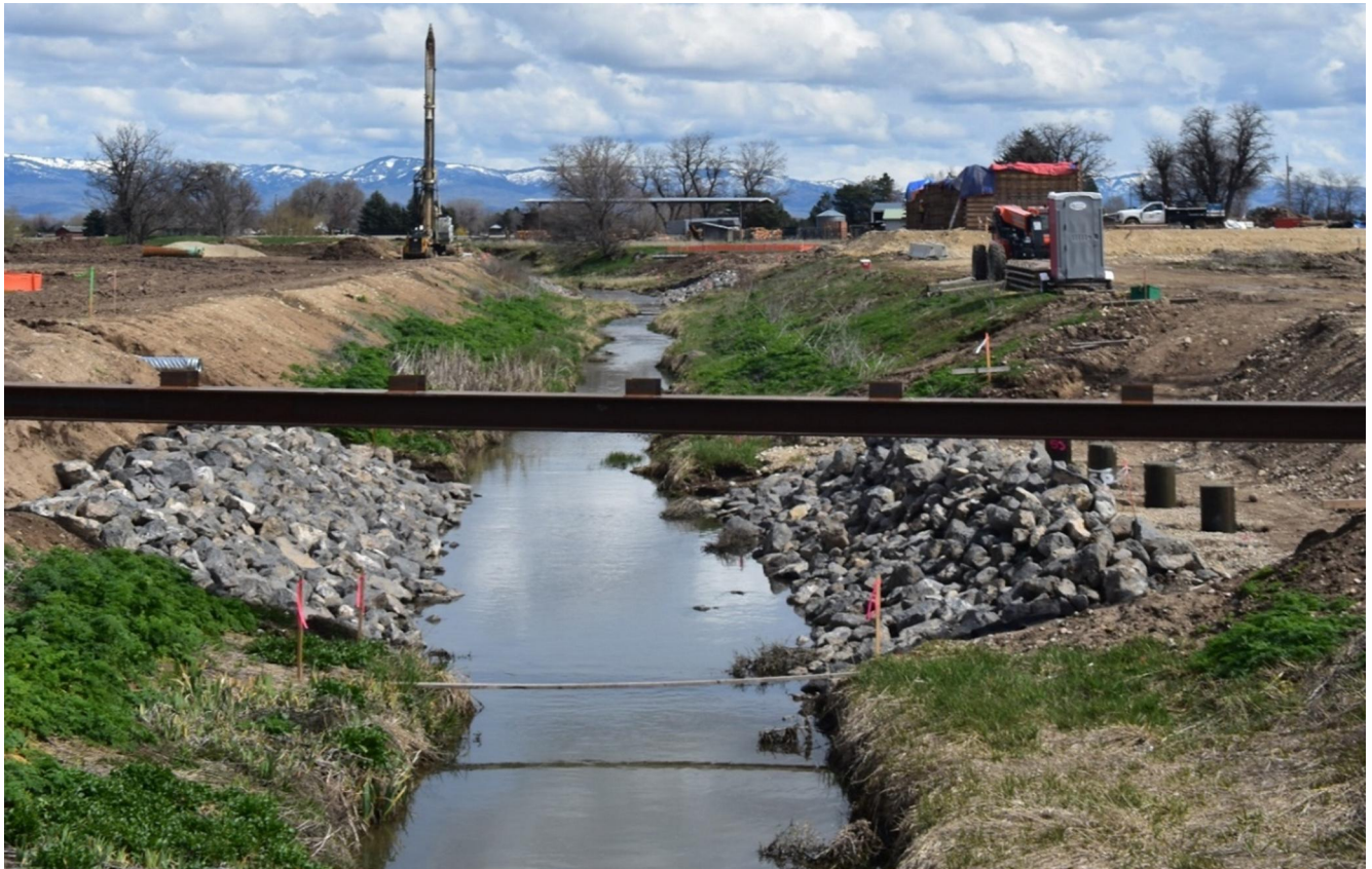
Figure 4 – SH-16/ Quasi Place Bridge Location (Looking East)
