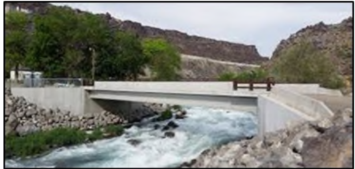
Example of Concrete Deck Bulb-Tee Bridge
