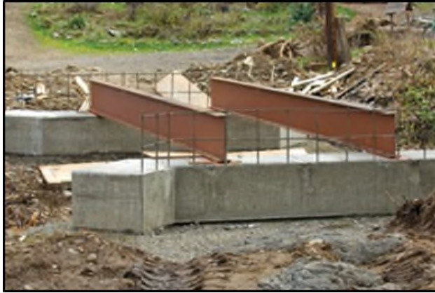
Example of Steel Plate Girder Bridge Construction (left) and Final Product (right)
