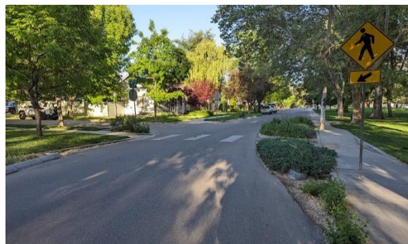
Chicanes in Boise: Chicanes are an alternating series of curb extensions along a roadway. They make drivers follow a curving pattern and discourage speeding. Quick-build options for chicanes may include bollards, planters, or materials with vertical separation.
