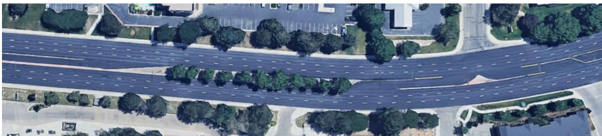
Raised Medians and Channelization on Parkcenter Boulevard in Boise: This treatment restricts left-turns from and channelized left-turns to adjacent side streets. Raised medians with larger buffer areas can provide a greater deterrent and are more visible than extruded curbs or other temporary treatments access management treatments. (Source: Google Maps)
