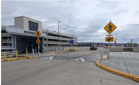
Example of Raised Crossing at Boise Airport: Raised crossings can increase awareness for drivers approaching a crossing and provide traffic calming benefits along a corridor, especially when placed at mid-block locations between roundabouts other traffic control devices. (Source: Google Maps)
