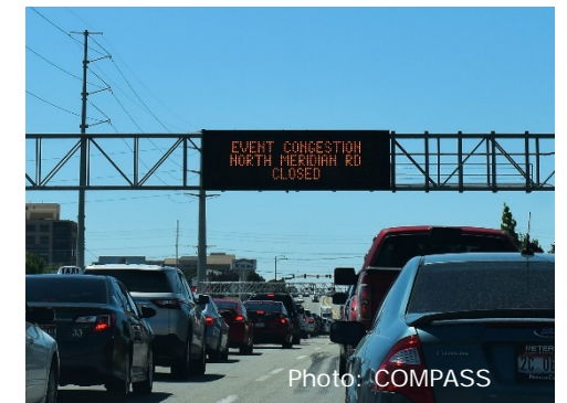
Photo: COMPASS Digital message boards make drivers aware of upcoming conditions and provide other relevant information.
