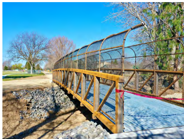
Figure 4: Cassia Street Bikeway and Sidewalk Project. The new Cassia Park Bridge provides critical connection over irrigation canal for Cassia Street multi-use path.
