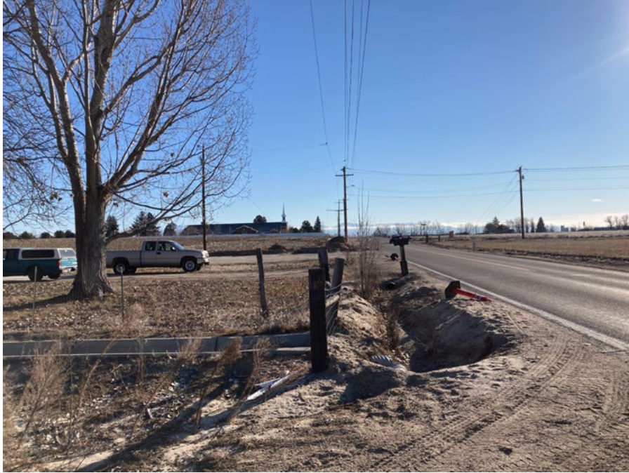
Floating Feather Rd, looking east: irrigation channel; private fence relocation; ROW acquisition
