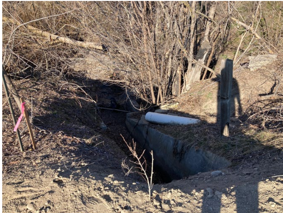
Alternative A at Foothill Ditch, looking west: steep embankment and culvert outlet
