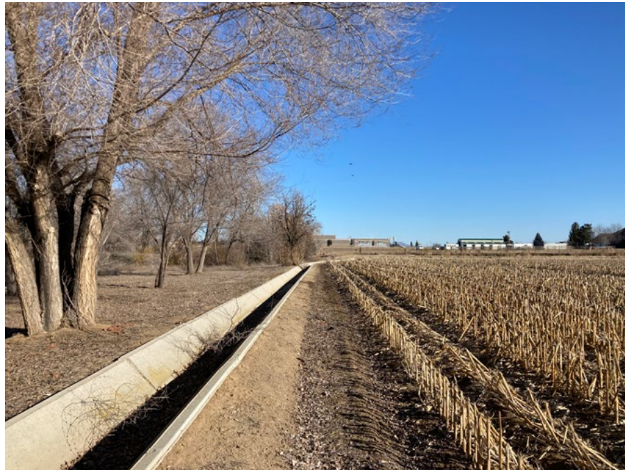
Alternative A, looking north: adjacent irrigation channel
