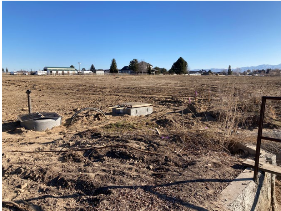
North of Foothill Ditch and east of Alternative A alignment: dead end system vaults, newly constructed for private development
