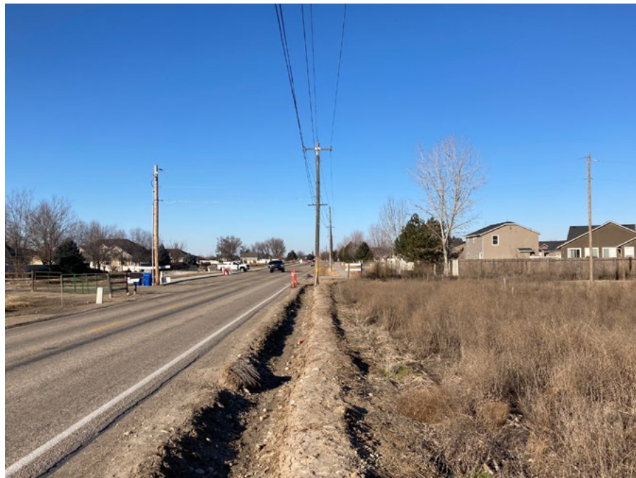
Floating Feather Rd, looking west: irrigation channel and utility poles; to continue existing sidewalk alignment, 4-6' of ROW acquisition likely
