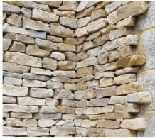
stone wall cladding
