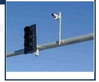
**Project Description:** Install upgraded signal controllers and radar detection at signalized intersections along the SH-55 (Eagle Road) corridor that ties into ACHD's Signal Performance Measure software. The Signal Performance Measure software provides a visual display of traffic data to aid engineers in signal timing and coordination and assist technicians with better responsiveness for maintenance of field hardware.
