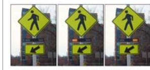
Figure 1. Example of an RRFB (left) and illuminated during the flash period (center and right) combined with W11-2 sign and W16-7P plaque at an uncontrolled marked crosswalk.
