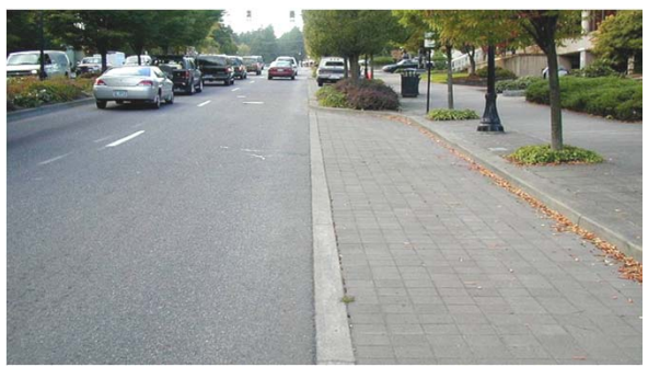
After: curb extension integral to sidewalk Street looks narrow even with no parked cars
