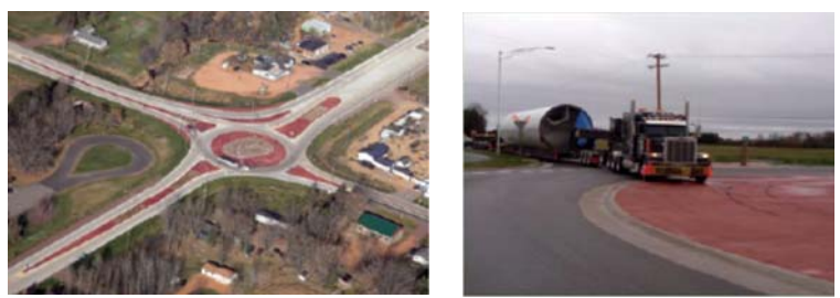
A Roundabout with Space for Over-size Trucks
