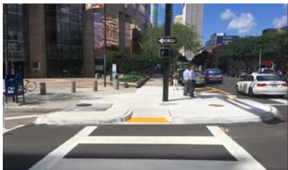
• Curb extension retrofit
